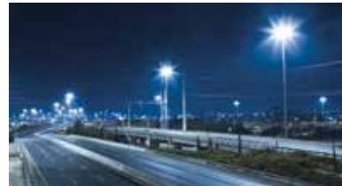
Connection of street lighting LED Luminaires (Rome, Italy). Series TH405.
